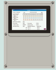
PAW-A2W-CMH Cascade Controller. Modbus IP for BMS communication.
